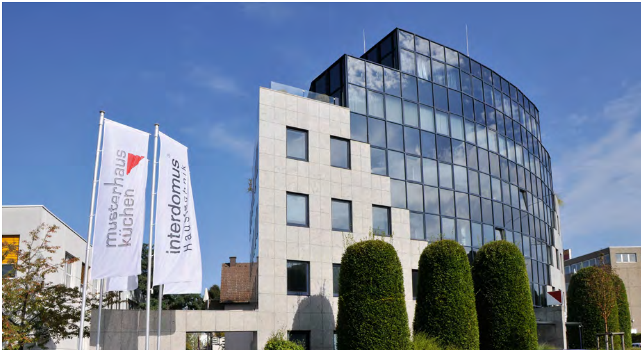
MHK headquarters in Dreieich
